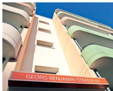
Renovated apartment complex: new cityscape – new attitude towards life
